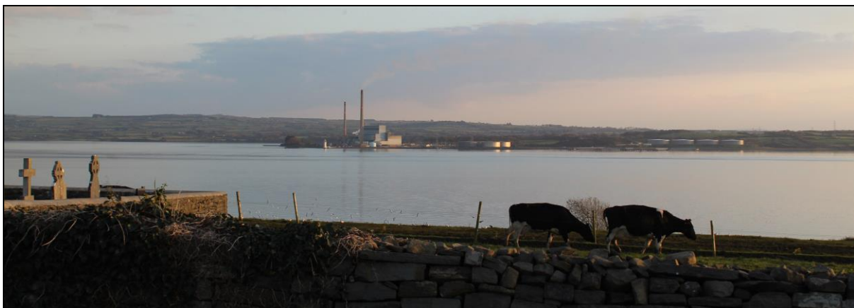
Plate 13.1: View of Shannon Estuary, the North Kerry coastline and Tarbert power station
